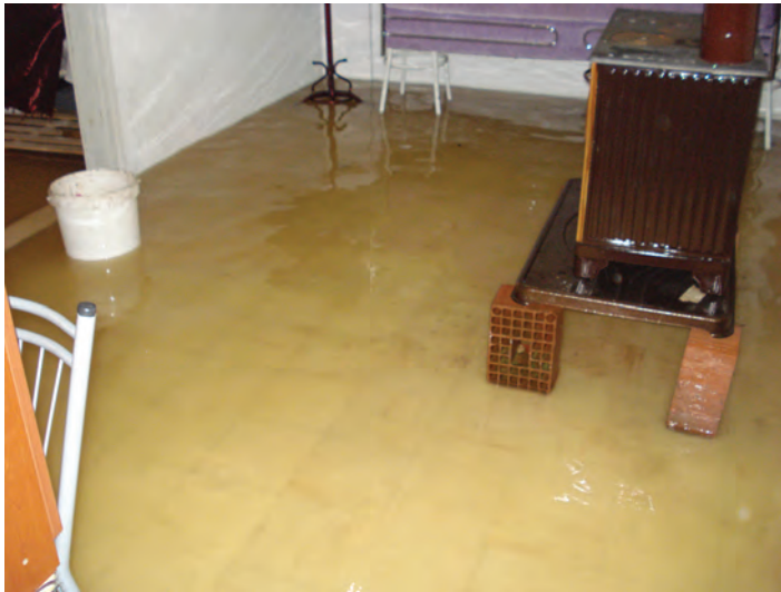
PHOTO 4 Affected house in Panayır
